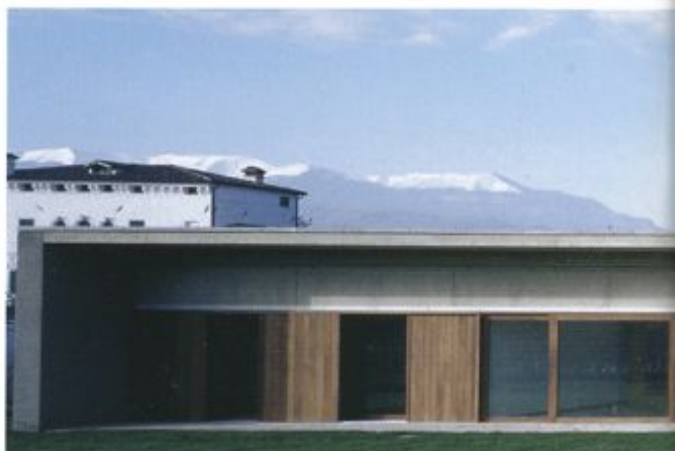
Teaching spaces line the openings formed by the two concrete enclosures, inset slightly and lined with gravel as thresholds to the adjoining landscape – communal spaces are identified with the rust-red roof profile above.
