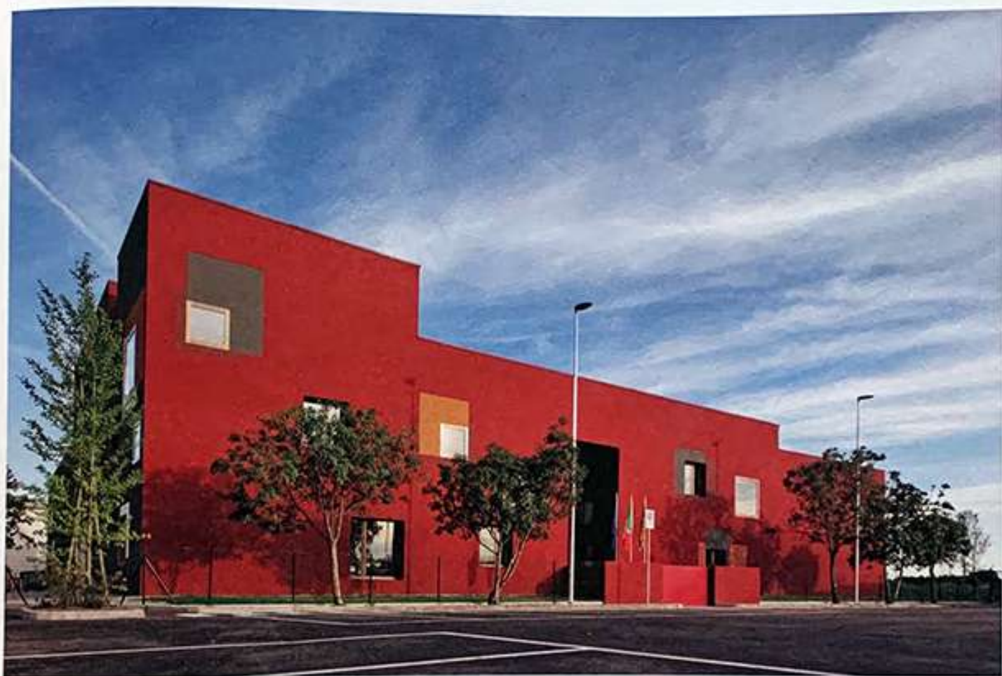
The plastered, bright red and anthracite grey facades are reminiscent of the traditional country estates of Veneto, creating a link with the regional building culture.
