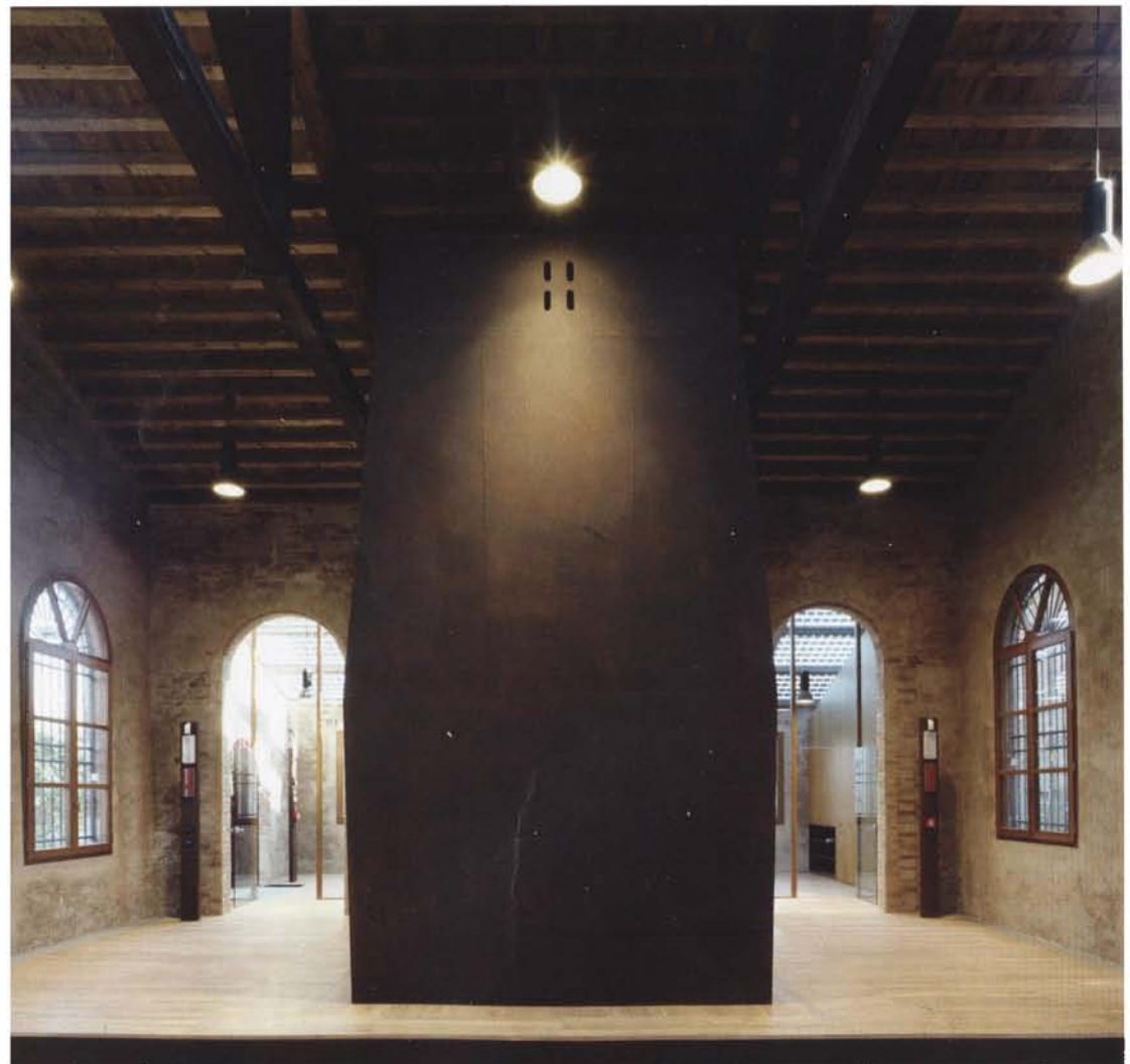
↑ By keeping the interventions to a minimum, the building retains its original quality. ↓ Cor-Ten steel box containing all services
